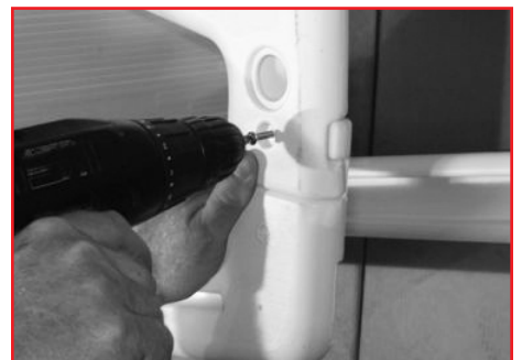
#5: Connect the top of the rails together using one #10 x 1-1/4" self tapping screw.
