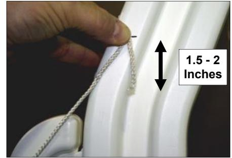
**Step 4: Make sure gate latch catch is in down / locked position over striker bar. Extend string upwards to outside face of upper handrail & fold end approx. 1.5 - 2 inches. Mark handrail at fold in string for location of eye screw (see also Step 5 below)**
