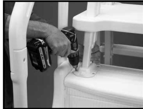
**#4:** Position the ladder over the pool step with the Mounting Blocks sitting flat on the top tread. Center the ladder side-to-side and align the back of the Mounting Blocks next to the groove in the back of the Platform as shown. Attach using four #10 x 3/4" self-tapping screws in each Mounting Block.
