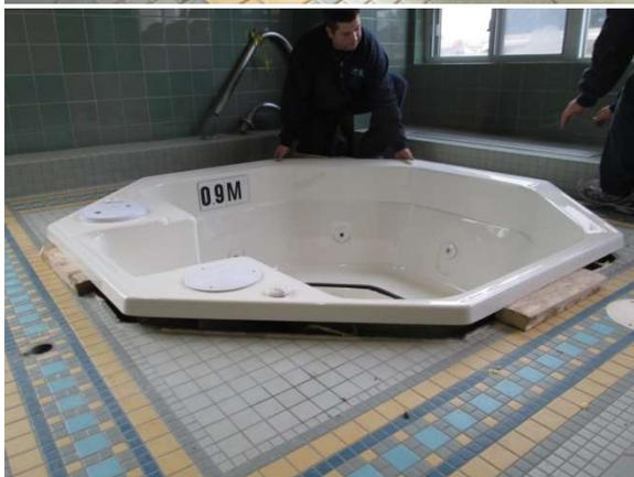
Once all final finishing of the floor around the hot tub is completed a bead of silicone should be placed around the outside bottom edge of the tub. This is to prevent any excess water in the surrounding area from going into the pad.
