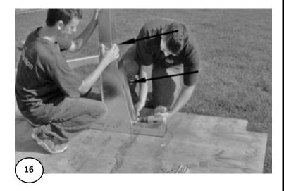
g. In order to ensure that the steel upright and the channels are at right angles during the assembly, push the ends of the steel upright and the channels and tighten the bolts at the same time. First, tighten the bolts of the channels by maintaining a good pressure. For the screws on the steel upright and gussets, sufficiently tighten the bolts to let the screws exceed 1/8". (Images 17 & 18)
