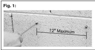
be no further apart than twelve (12) inches. Do not tighten screws all the way. (Fig. 1)
