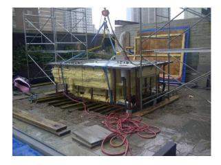
Prior to lowering the hot tub, place long 1" thick pieces of wood around the sides of the pad. Lower the tub onto the wooden beams. This will allow you to easily shift the tub to straighten it. Once this is complete you can remove the beams.
