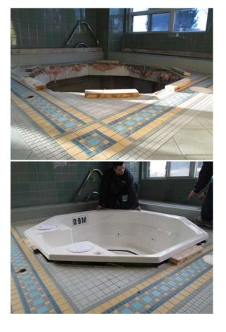
Once all final finishing of the floor around the hot tub is completed a bead of silicone should be placed around the outside bottom edge of the tub. This is to prevent any excess water in the surrounding area from going into the pad.
